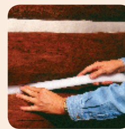
1. Start with logs that are stained with a coating compatible to Log Jam® and have properly installed backer material.
