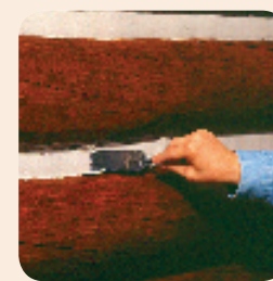
5. Tool to ensure a tight seal to the top and bottom of the chink line.
