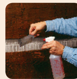
4. Lightly mist the trowel as needed.
