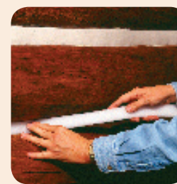
1. Install Grip Strip into caulk well of clean, stained logs.
