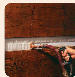
3. Gun Log Jam® over the backer material.
