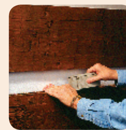
2. Tape the entire joint using polyester tape.
