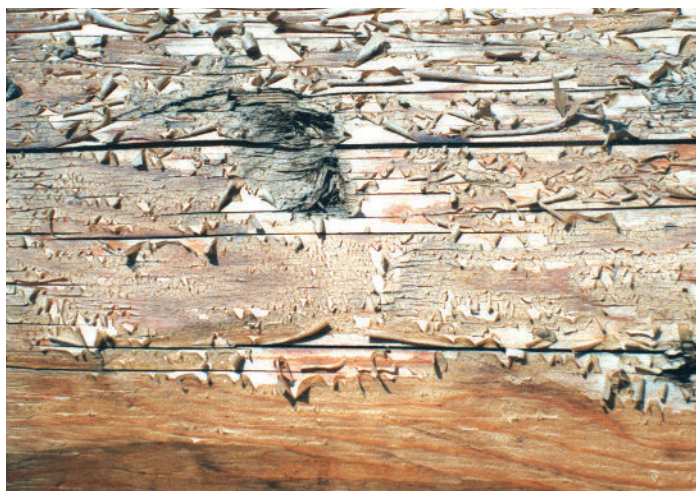
Too much water vapor pressure can result in stain that peels, as pictured.
