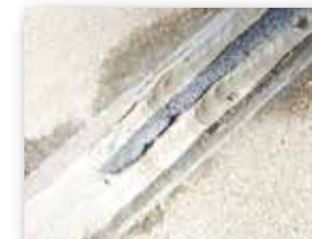
WIDE CRACK: Apply 3 beads of caulk (edges first, center bead last)
