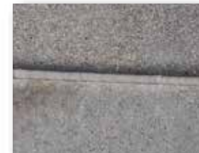
NARROW CRACK: Apply 1 bead of caulk
