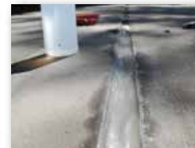
Slightly recessed Slab bead after cure
